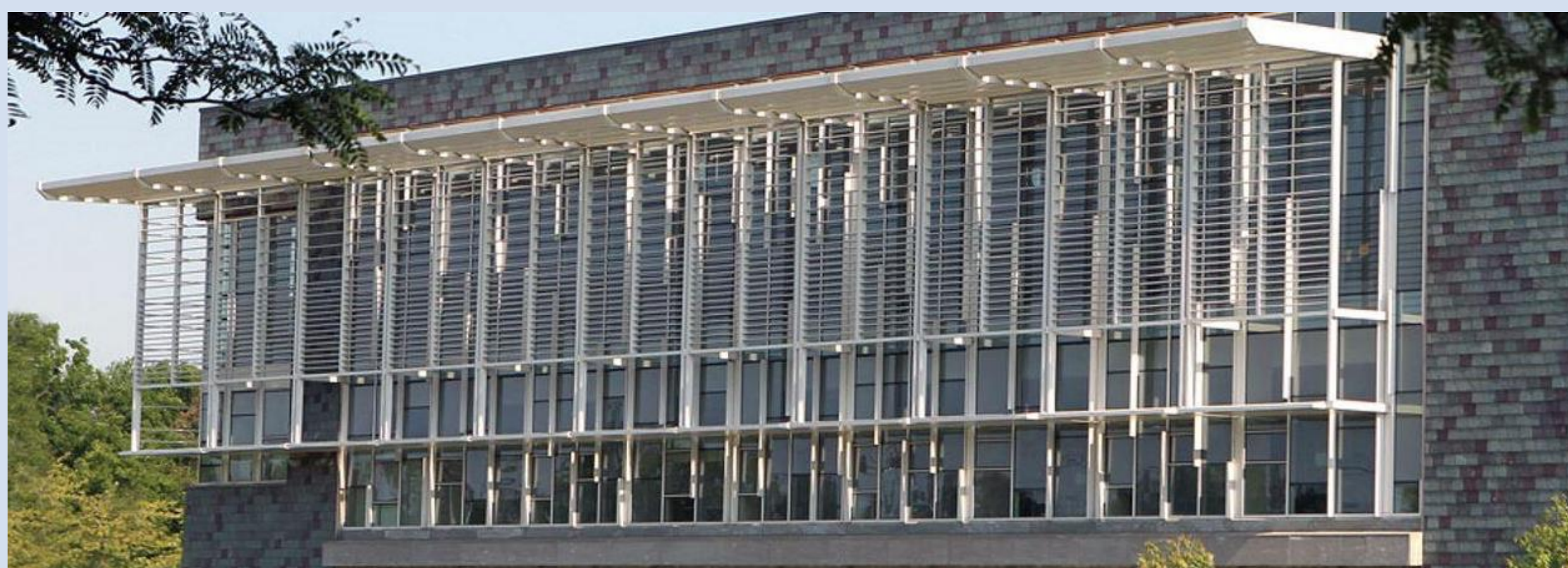
Figure 1. RIC façade-controls amount of sunlight heating the building.
