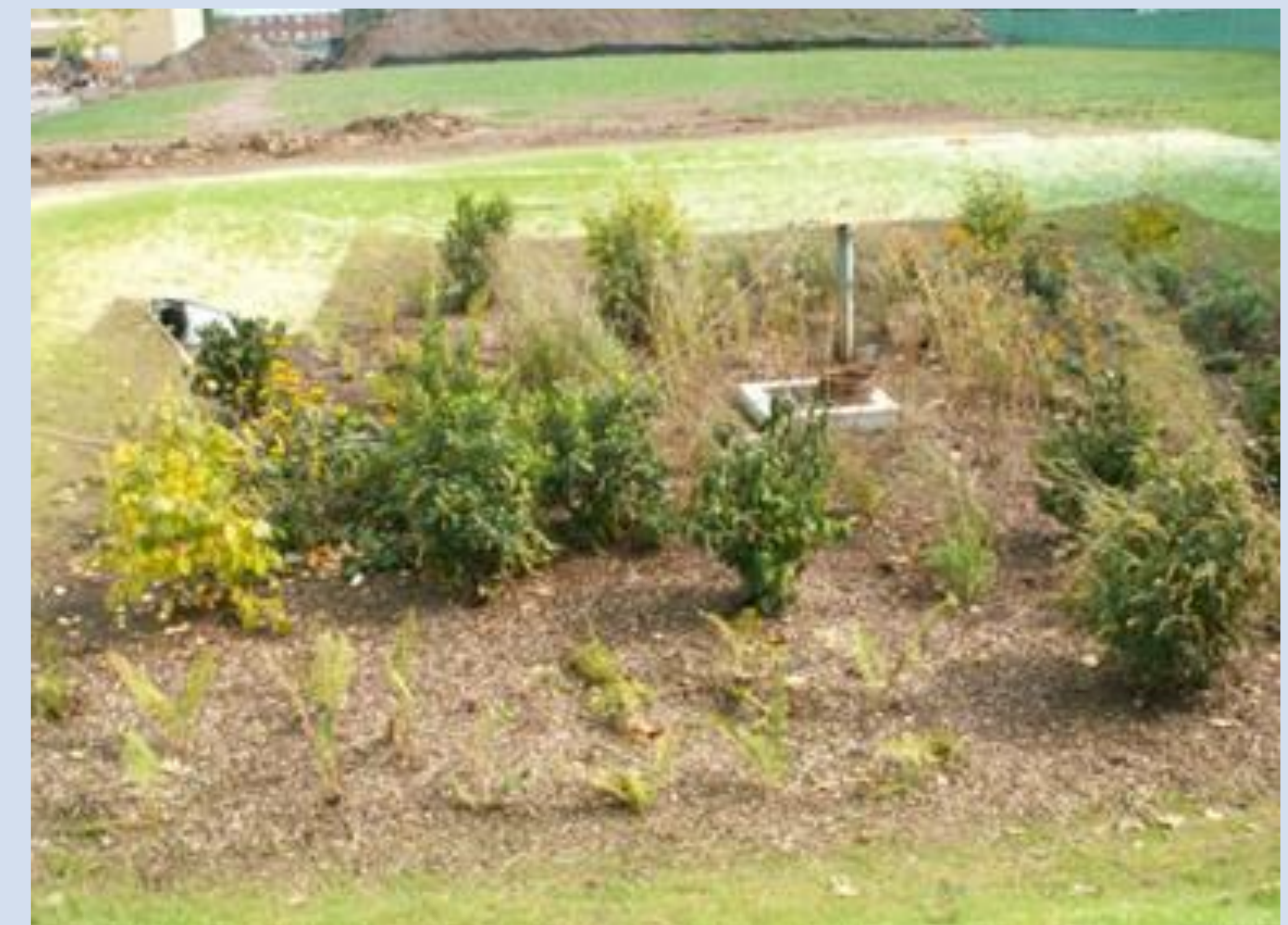
Figure 4. Bioswale helps to improve stormwater control and purify water.
